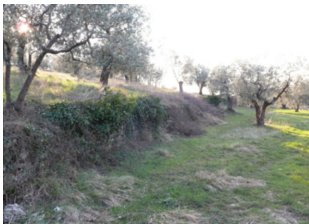
Figure 8. Example of a stone wall almost totally collapsed. Although they are degraded, terraces still maintain a residual function on soil erosion control (Prato, Tuscany).
