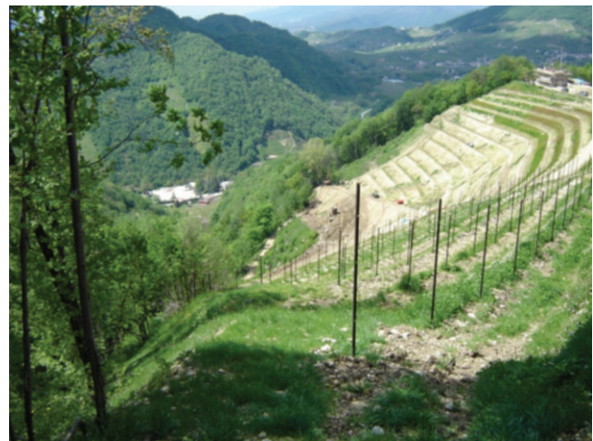
Figure 1. Earth terraces under construction in Veneto (in the Prosecco wine area).
