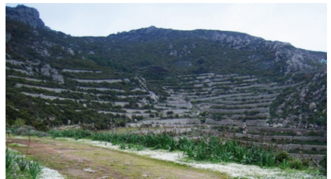
Figure 6. Stonewall terraces set up on compact bedrock at Capraia isle (Tyrrhenian sea) with shrubs and forest in evolution. Terraces were built by prisoners before the dismissing of the penitentiary. In this case the abandonment of agriculture did not lead to degradation of terraces. (Image by Andrea Gervasoni, 2009).
