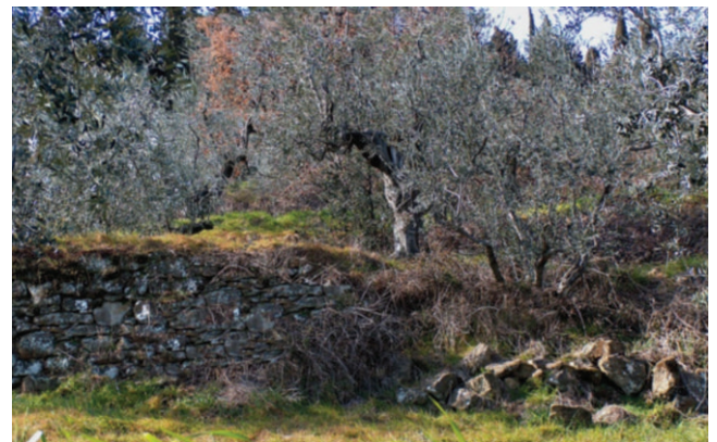
Figure 7. Stone wall terraces set up on incoherent colluvium (Fiesole, Tuscany). Agriculture is almost abandoned and degradation of terraces is going on, but the slope gradient of terraces is still sufficiently conserved.
